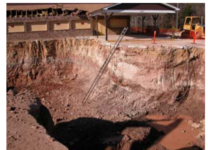
Dispenser Island Excavation
